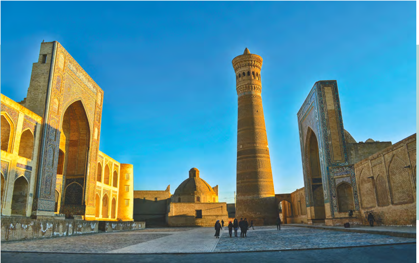
Ensemble Poi-Kalon, Bukhara
